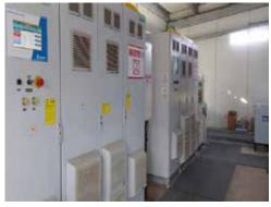
Plate 7. Inverter Rooms converting DC power from Solar Panels to AC, with real time monitoring
