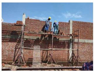
Figure 10 - Image showing the construction of the compound wall (Source: CSCL)
