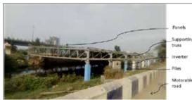
Fig. 3. View of the panels from top (Banerjee, 2021) Fig.4. View from the canal side road of of the installed 500kW solar PV plant parts Source: Author
